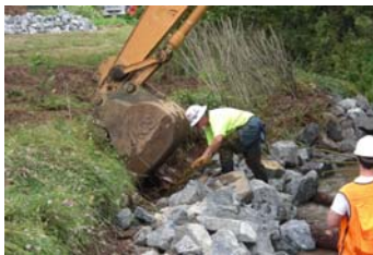
June 2009: Dave Derrick installing willow cuttings with use of yellow machine above LPSTP
